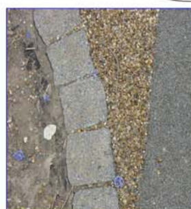
The gravel paving has chips stuck down. Water can go through it when it rains. This is good for the trees.
